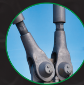
Cable Tensioner - Post Tension System
